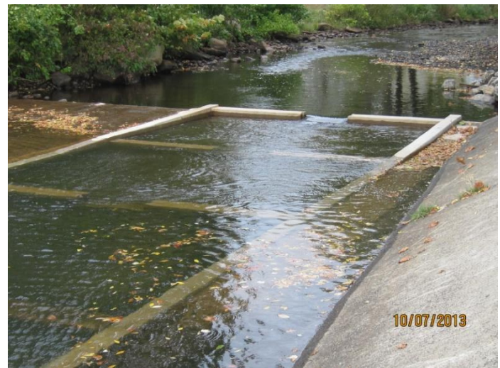
Pequonnock River Apron Fishway: The five-pool pool-and-weir fishway is mostly underwater during high tide but there are drops at each weir during low tide. More photos of this fishway later.
