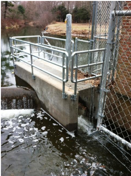
East Haven Diversion Dam Fishway: Even a small dam like this can block runs of river herring. Instead the concrete 'box' is one section of steep pass fishway. To the right is a brick gatehouse.
